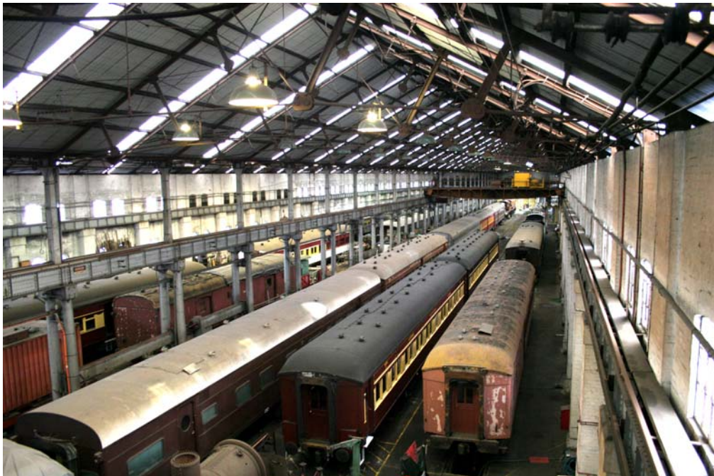
Inside the Large Erecting Shop
